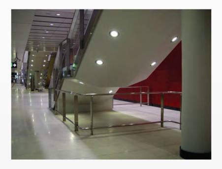
Figure 175: Detectable Barrier
