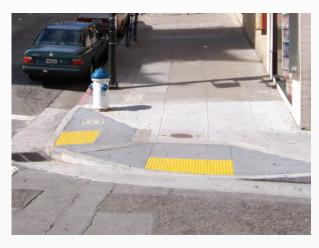
Figure 215: Detectable Warning Surface at Kerb cut
