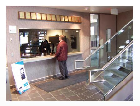
Figure 176: Detectable Handrail
