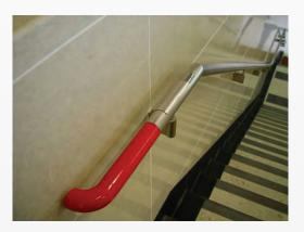
Figure 202: Handrail Extensions
