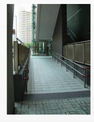
Figure 203: Dual Height Handrails
