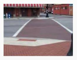
Figure 56: Detectable Warning Surfaces
