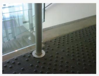
Figure 216: Detectable Warning Surface at Top of Stair
