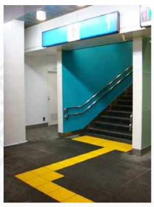
Figure 92. Tactile Guideway Consisting of Truncated Domes along Complex Path to a Known Destination (e.g. stairway) - Source: UDA & Associates, Canada
