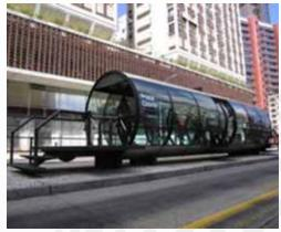
Figure 93. A BRT Stop in Curitiba, Brazil with Sliding Doors
