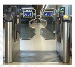
Figure 94. Access Gate Designed to Accommodate Mobility Aid
