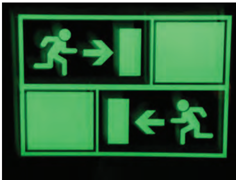
Figure 93: Illuminated emergency route sign at night
