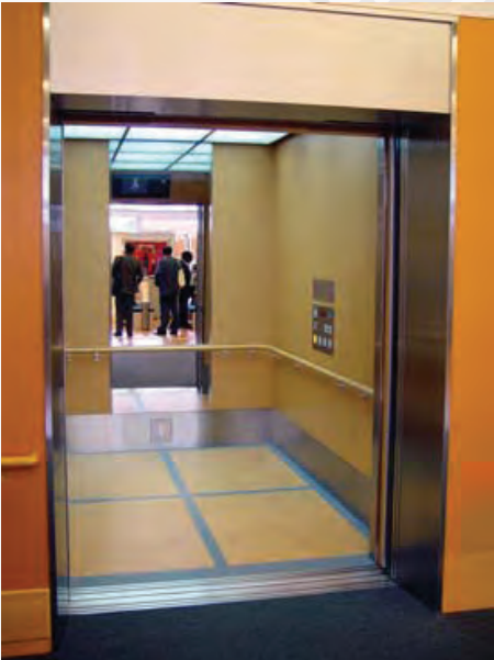
Figure 147: Elevator showing an example of lowered and large interior call buttons, and colour definition on the floor.
