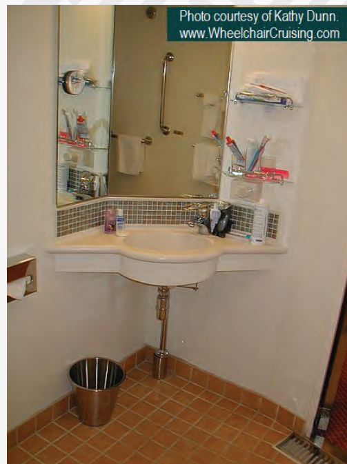
Figure 111: Accessible cabin's roll-under hand basin (Source: Princess Cruises: Island Princess, from website http://www.wheelchaircruising.com/princess.html accessed 20/08/09)
