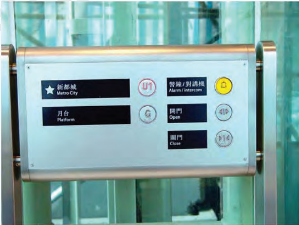
Figure 148: An example of an elevator control panel featuring colour contrast and tactile bilingual text, buttons and symbols.
