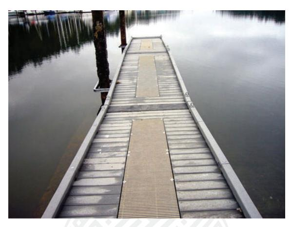
Figure 65: An example of using gentle ramping to allow the maximum number of users to gain access. Ideally, provision should be made for some form of guard or protection rail to prevent persons on the quay from falling into the water.
