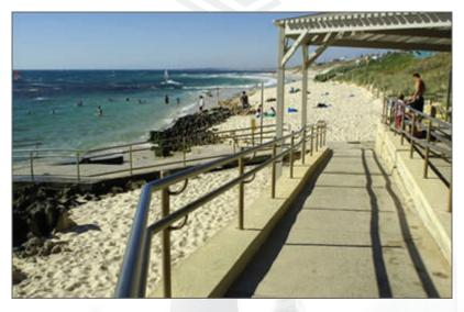
Figure 76. An example of the usage of ramping to achieve access to beach surfaces. This particular example illustrates an important principle within the framework of universal access, namely achieving accessibility on the main circulation path instead of specialized provision.
