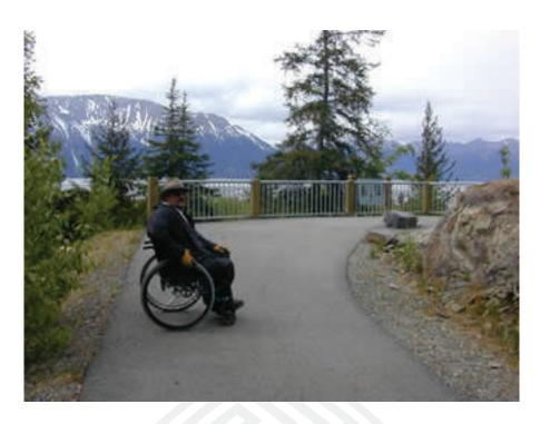
Figure 75. This image clearly illustrates the methods in which the usability of vistas, overlooks and exterior areas can be designed in a manner allowing the maximum feasible physical accessibility. Note, in particular, the usage of clear protective devices, which physically prevent harm, the clear distinction between environment and path, as well as the nature of the pathway surface itself.
