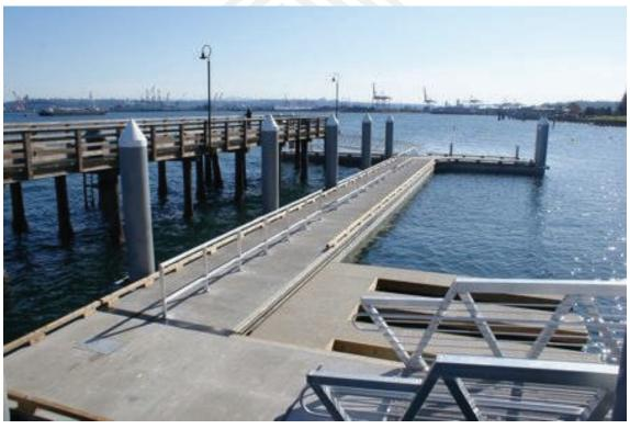
Figure 90. This illustration indicates some of the features that may contribute to creating access: almost level throughsurfaces, ramped access across different heights, railings to designate ends of platforms and flexible junctions. [Source: http://westseattleblog.com/blog/wp-content/uploads/2010/03/gangwaysouther.jpg]
