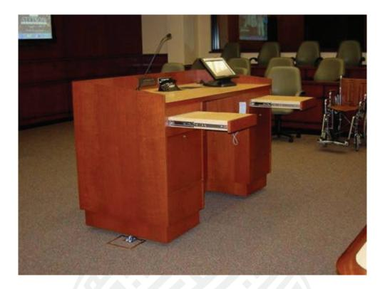
Figure 35. Accessible lectern with knee and toe clearance [Source: http://www.access-board.gov/caac/report\_clip\_image002\_0027.jpg]
