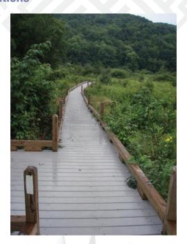
Figure 72. Level gangways provide wheeled users, and persons with difficulty walking, with opportunities to access hiking and trail experiences. The usage of lowered portions prevents wheels from slipping over gangway ends, as well as providing a mechanism for persons with functional visual limitations to detect and react accordingly, to gangway edges.
