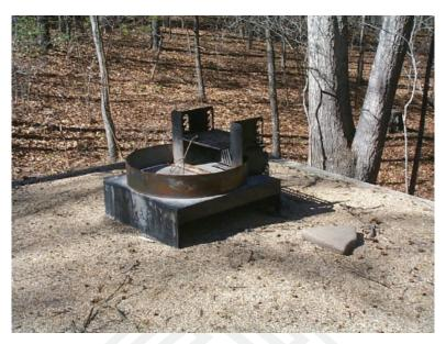
Figure 83. A fire-ring built in a manner such that physical access may be gained. Note the raising of the ring above the ground, which provides both safety for children and other users, as well as ensuring that persons with functional visual limitations are able to detect the position of the fire-ring.
